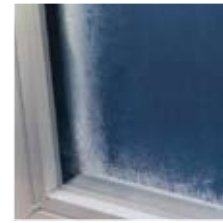
Less-Metal Spacer Mid-performance spacer systems improve condensation resistance.
