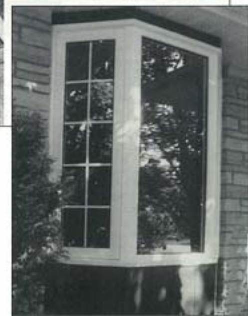
Muntin bar assembly (above) for use in Georgian bay-windows.
