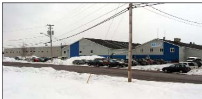
Atlantic manufactures from three buildings, totaling 105,000 square feet
