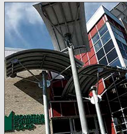
MEC's Winnipeg store uses approximately 47% less energy than the baseline specified in the federal government's model energy code for buildings. It reduces greenhouse gas emissions by more than 30 tons per year compared to conventional buildings and was built using 97% recycled materials.
