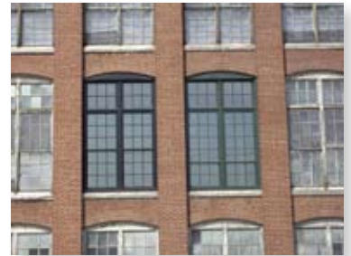
Before and After: Installed 700 Series units in Langston Terrace Dwellings restoration project
